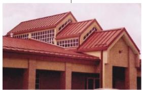
Metal roofing is available in both structural (low- and steep-slope) and architectural applications. Both curb appeal and exceptional performance are an owner's goal for any system, according to TMI, with the coalition noting a growing trend toward steeper slopes and overstated, extended, or molded roof fascias.
