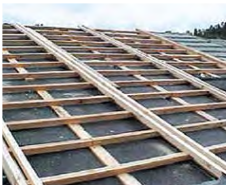
Fig 1: Batten and Counter-batten system used to mount stone-coated metal roofs
