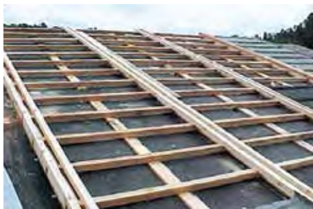
Fig 1: Batten and Counter-batten system used to mount stone-coated metal roofs
