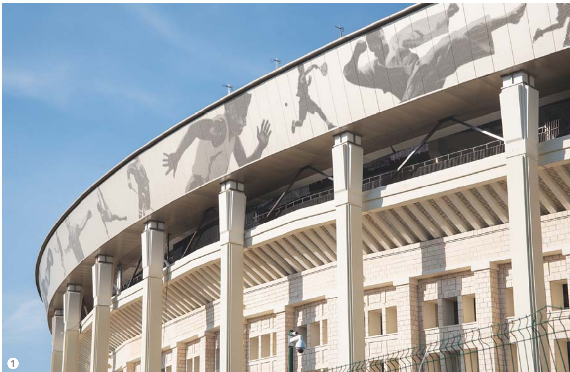
Figure 1: Detail of the Luzhniki Stadium, painted with PVDF products supplied by Salchi Metalcoat.
